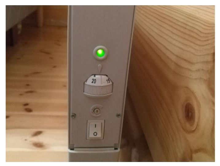
Instead of sliders there is a knob. The arrow should be set to minimum 15 and maximum 22 degrees. When Alex turns on the preservation mode, the system will reset the temperature 10 degrees.
