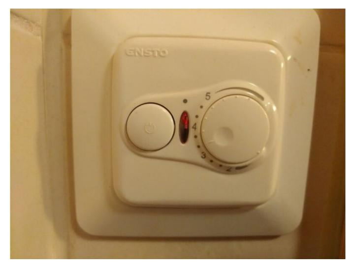
The floor heating must be always ON and in position "2".
